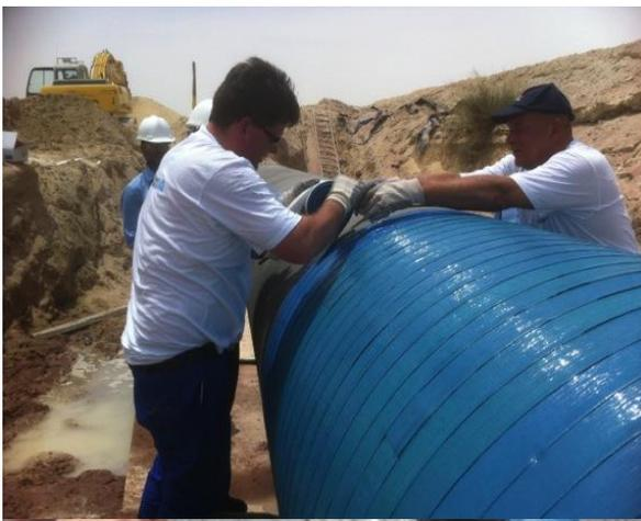
Fig. 1 Application of VEC's at a 48 inch pipeline in Sabkha area
