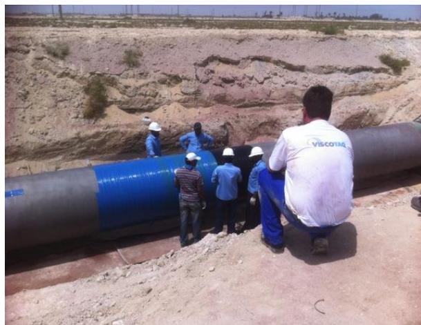
Fig. 2 Application of protective outer layer
